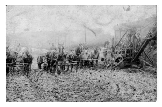
A great photo of construction on the National Road (which would become U.S. Rt. 40 when the U.S. Highway System began in 1926) at Bridgeport, Ohio in Belmont County. This photo was from 1918 when the highway section between Bridgeport and Cambridge first being paved with bricks; other sections of this highway would follow with paving in the upcoming years. (This is from OLD PHOTOS SOUTHERN OHIO a public Facebook page.)
